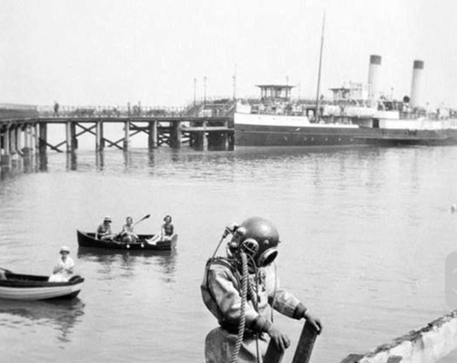
t the end of the 1920s, the effects of the gribble worm were beginning to be seen on the structure of both Piers. This tiny little crustacean burrows into the wood of the piles gradually destroying them. The Pier master at the time had to be a hard hat diver and was responsible for encasing the damaged piles in concrete.
